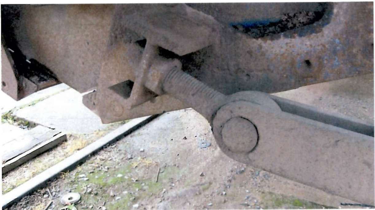
Figure 5 – close up of detail
