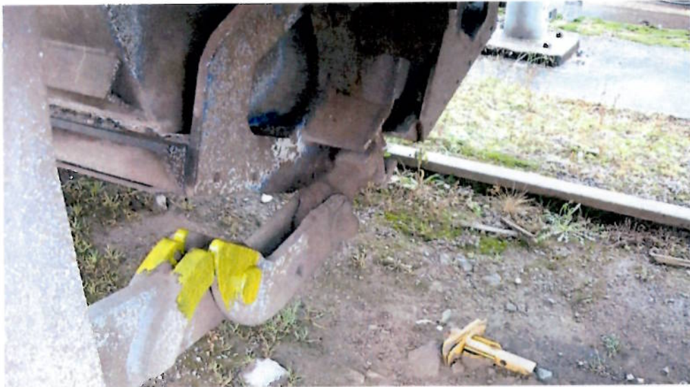
Figure 4 – example of an eyebolt in situ.
